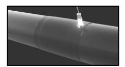
4. Remove protecting foil from the sleeve and move the sleeve along the jacket pipe to a position between the marks made earlier at step
