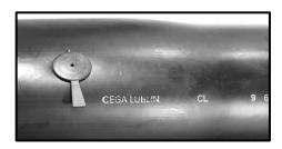
13. Immediately after filling the PUR into the holes, the holes shall be bunged by impaling the venting plugs. The plugs shall be placed in a way that their "tales" are perpendicularly to the axis of the pipe.
