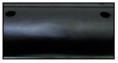
10. Make two filling holes in the top of the sleeve by using driller  $\emptyset$ 24mm.
