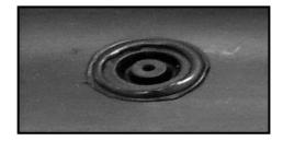
15. Install the welding plugs according to instruction of the welding unit. Parallel heating up of one of the hole and one of the plug for 30 sec with  $230^{\circ}C$  of the heater, and later regular pressing of the plug up to the cooling down of this joint is recommended. Repeat this operation with the second filling hole and plug.
