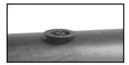
14. The venting plugs shall be removed after degassing and cooling down of the PUR foam and the sleeve, than if needed the filling holes shall be broached up to Ø24 mm to enable installation of the welding plugs.
