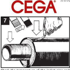
Check the temperature of the jacket pipe and the service pipe with the temperature indicator. An immediate change of its color means the correct temperature has been reached. The pyrometer can also be used for checking of the temperature.
