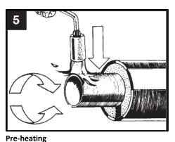
Pre-heat the service pipe first 60°C, avoid direct contact between flame and the foam.
