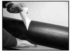
6. Remove the foil protecting the mastic sealing strip from inside the sleeve.
