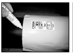
1. Place the sleeve centrally on the connected pre-insulated pipe. Mark both ends of the sleeve around on the surface of the jacket pipe. Move the sleeve on side along the jacket pipe for a distance allowing to prepare the installation space.
