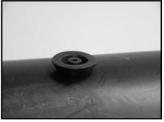
**12.** After degassing and cooling down of the PUR foam and the sleeve, the venting plugs shall be removed, than if needed the filling holes shall be reamered up to Ø24 mm to enable installation of the welding plugs.
