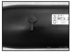
**11.** Immediately after filling in of the PUR, the holes shall be bunged by impaling the venting plugs. The plugs shall be placed in a way that their "tales" are perpendicularly to the axis of the pipe.
