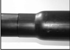
**8**. The surface of the sleeve shall be soft but not scorched. Soon minor efflux of the mastic shall be seen around the ends of the sleeve.
