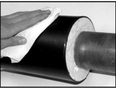
2. Clean the surface of the jacket pipe by the cleaning tissue with acetone or alcohol, remove any oil, grease etc. Activate the surface of the jacket pipe by tarnishing using the abrasive canvas (gr. 40-60)
