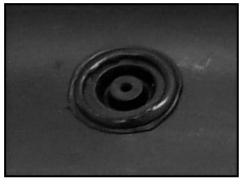
**13.** Install the welding plugs according to instruction of the welding unit. Parallel heating up of one of the filling hole and one plug for 30 seconds with  $230^{\circ}$ C of the heater, and later regular pressing of the plug up to the cooling down of this joint is recommended. Repeat above operation with the second filling hole and plug.
