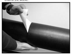
From inside the sleeve remove the foil protecting the mastic sealing strip.
