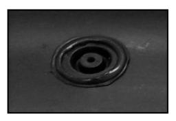
13. Install the welding plugs according to instruction of the welding unit. Parallel heating up of one of the filling hole and one of the plug for 30 sec with 230°C of the heater, and later regular pressing of the plug up to the cooling down of this joint is recommended. Repeat above operation with the second filling hole and plug.
