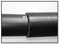
4. Remove the protecting foil from the sleeve and move the sleeve along the jacket pipe to a position between the marks made earlier at step
