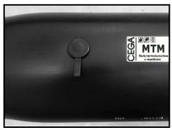
11. Immediately after filling the PUR into the holes, the holes shall be bunged by impaling the venting plugs. The plugs shall be placed in a way that their "tales" are perpendicularly to the axis of the pipe.
