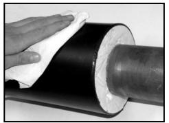
Clean the surface of the jacket pipe by the cloth with acetone or alcohol. Tarnish the surface of the jacket pipe by the abrasive canvas (gran.40-60).
