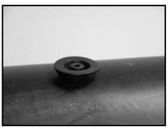
12. After degassing and cooling down of the PUR foam and the sleeve, the venting plugs shall be removed, than if needed the filling holes shall be reamered up to Ø24 mm to enable installation of the welding plugs.
