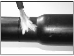
6. Start shrinking the sleeve on both of its ends. The soft yellow flame shall be used.
