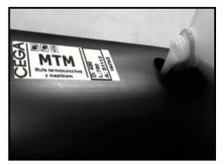
10. The PUR shall be filled into the sleeve through one of the filling holes.
