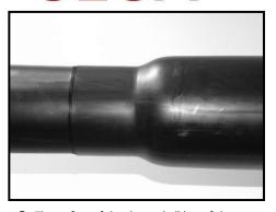
7. The surface of the sleeve shall be soft but not scorched. Soon minor efflux of the mastic shall be seen around the ends of the sleeve.
