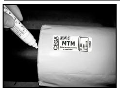
1. Put the sleeve centrally on the junction of the pre-insulated pipe. Mark both ends of the sleeve on the surface of the jacket pipe. Move the sleeve on side along the jacket pipe for a distance allowing to prepare the installation space.
